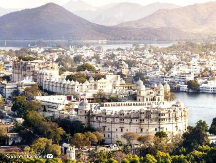
Picture 1 Aerial view of Udaipur's built heritage
